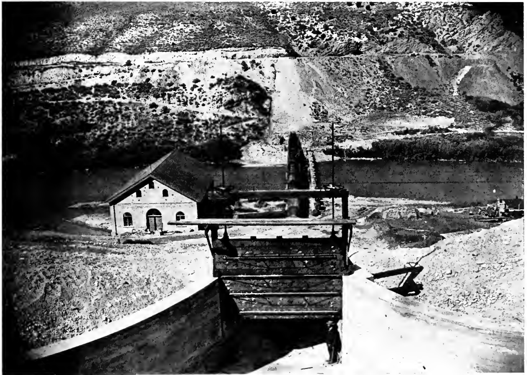
FIG. 1.—VIEW OF POWER HOUSE AND SIPHON SHOWING EAST INTAKE TO SIPHON PIPE.
